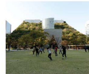
The ambient air temperature of the surrounding is reduced due to evapotranspiration of vegetation.
