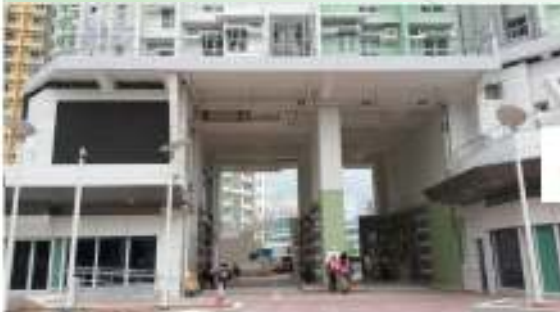
Ground Floor Ventilation Bays to enhance Wind Environment at Pedestrian Level
