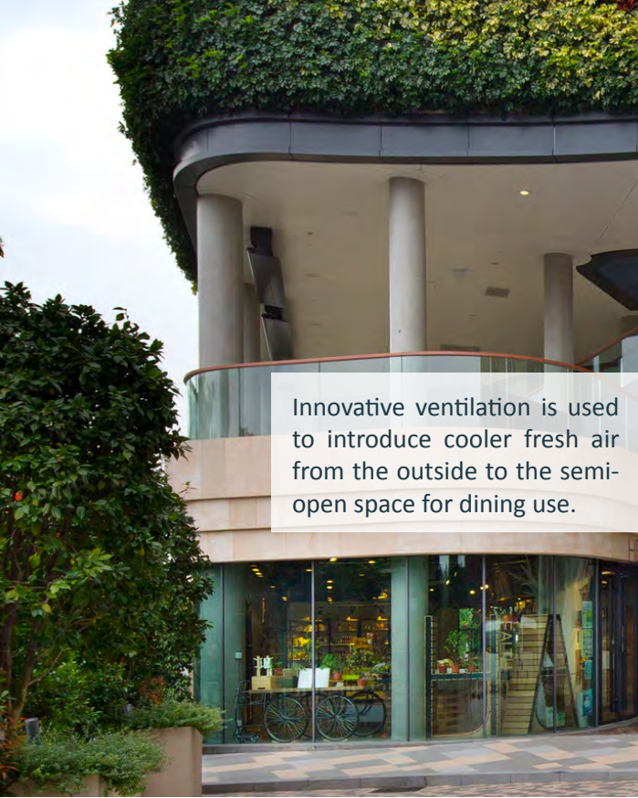
An extensive green wall with a leaf coverage of almost 100% helps reduce the façade surface and ambient air temperatures.
