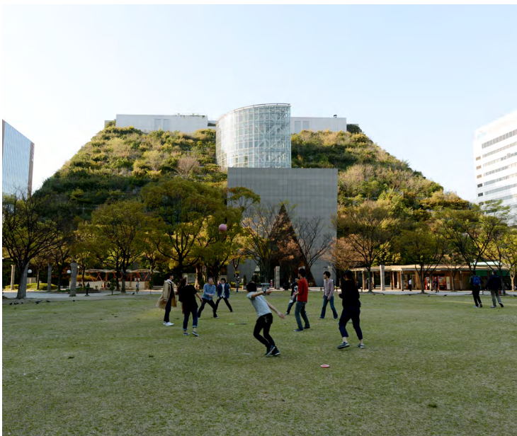
The ambient air temperature of the surrounding is reduced due to evapotranspiration of vegetation.
